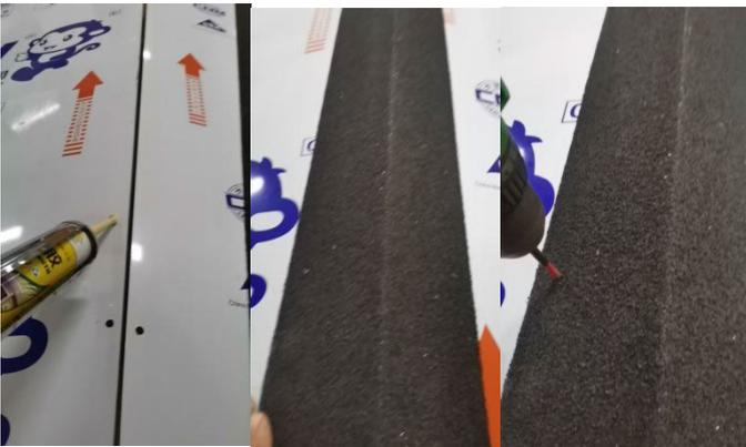
11. After assembly is finished, apply sealant to the areas shown below.
