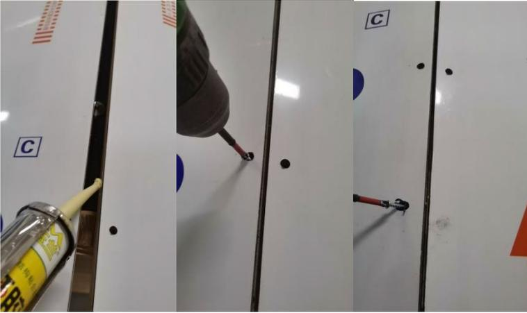
10. Apply sealant to the inside edges of the metal roof cover and secure it with screws.
